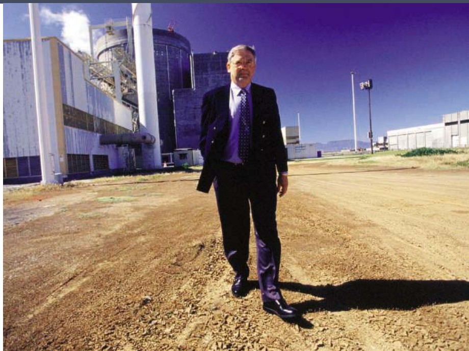
New ground. Pebble bed pioneer Dave Nicholls plans a new reactor here at Koeberg, South Africa.
